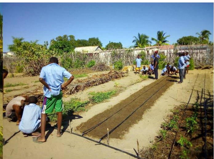
Installation of the micro-irrigation network by the students of the CEG of Saint- Augustin
